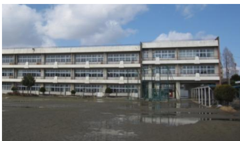
Figure 24. Settlement of school building in Osaki City
