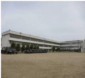
Figure 9. Overall view of damaged school building
