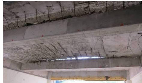
Figure 27. Slab uplifted and dismantled from beam
