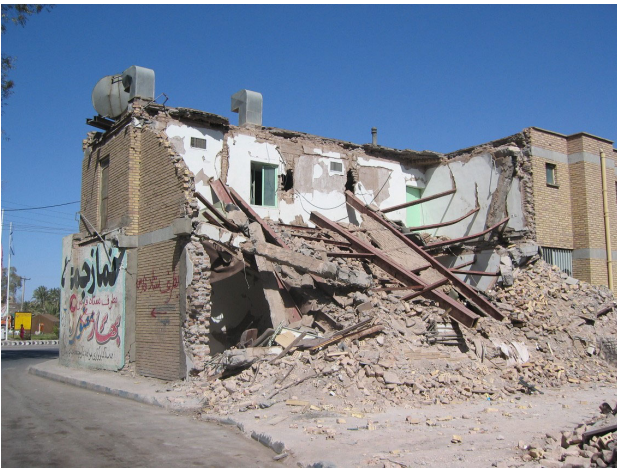
写真3 Governor's Building 南西角の崩壊
