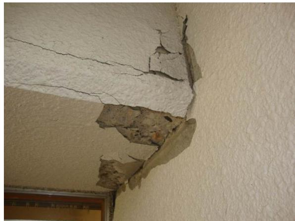
(d) Crush of concrete at plastic hinge region of a beam end
