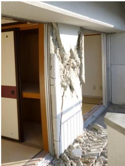
(c) Shear failure of non-structural wall
