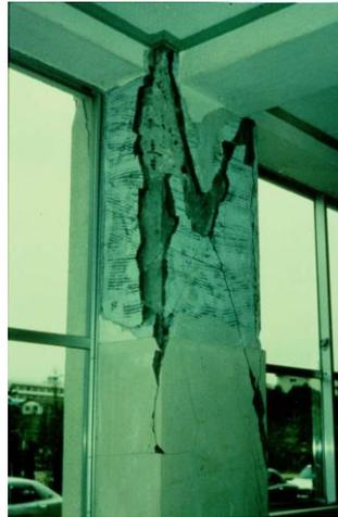
Damage class III: (left) Cracks with a width of about 2mm on structural concrete
