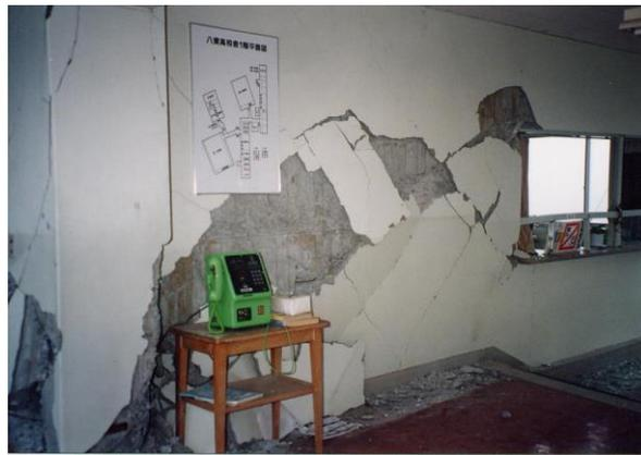
Damage class IV: Exposed rebars without buckling or fracture
