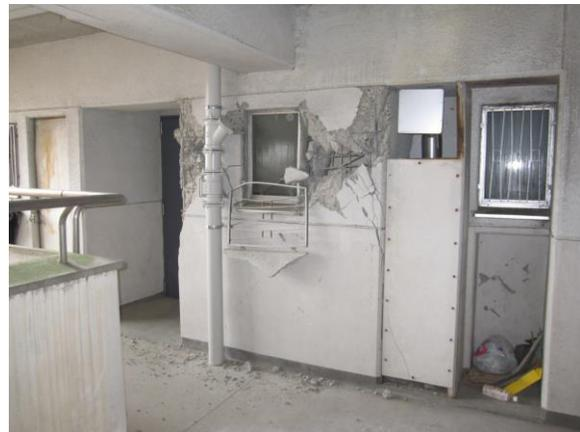
(b) Shear failure of non-structural wall
