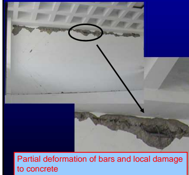
No buckling nor fracture of steel bars. Column sustains vertical load.
