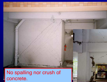
Some cracks at boundary of wall but no deformation of bars.
