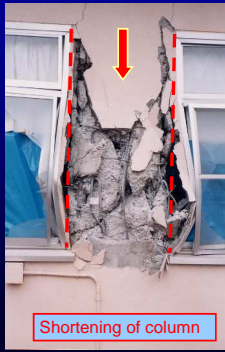
Large cracks and failure of concrete
