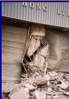
Shear failure (1995 Kobe EQ)
