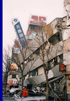
Collapse of RC buildings (1995 Kobe EQ)
