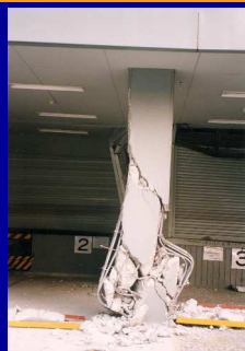
Shear failure (1995 Kobe EQ)
