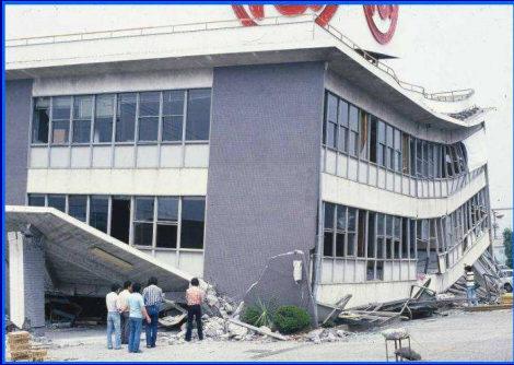
Collapse of buildings (1978 Miyagi-ken-oki EQ)
