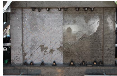
Fig.5–Damage at ultimate stage
