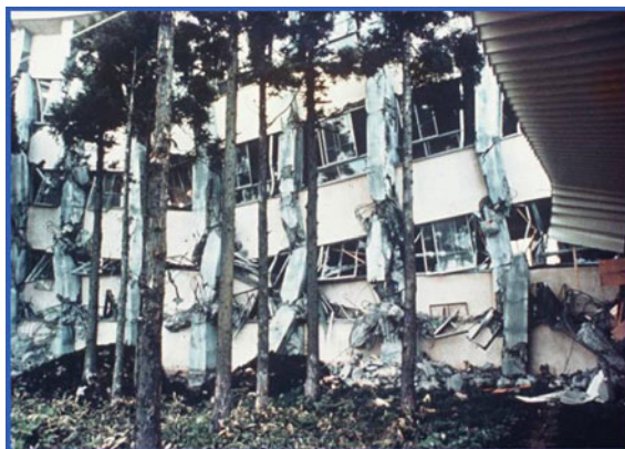
Fig. 1 Collapse of RC buildings in 1968 Tokachi-oki earthquake
