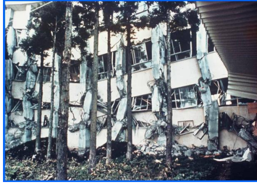
Fig. 1 - Collapse of RC buildings in 1968 Tokachi-oki Earthquake
