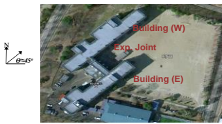
Fig.14 Three storied RC building
