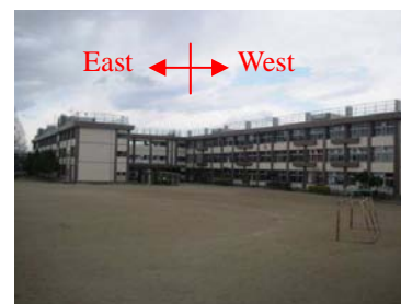
Fig.2 North view of H school building
